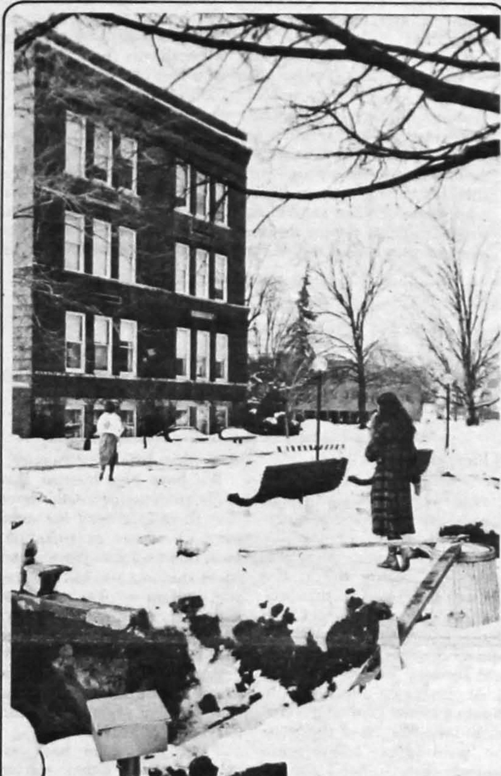
If temperatures continue to rise, Physical Plant personnel will soon be able to pour concrete anchors for the new steam heating pipe and cover up this ditch between the Administration and science buildings. The new pipe arrived late, causing the Physical Plant to "get caught by bad weather."
